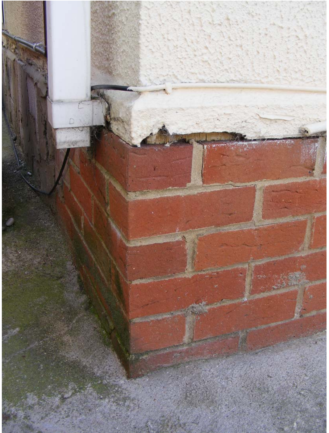
Brick plinths have been built to close the chassis and cover propped corners
