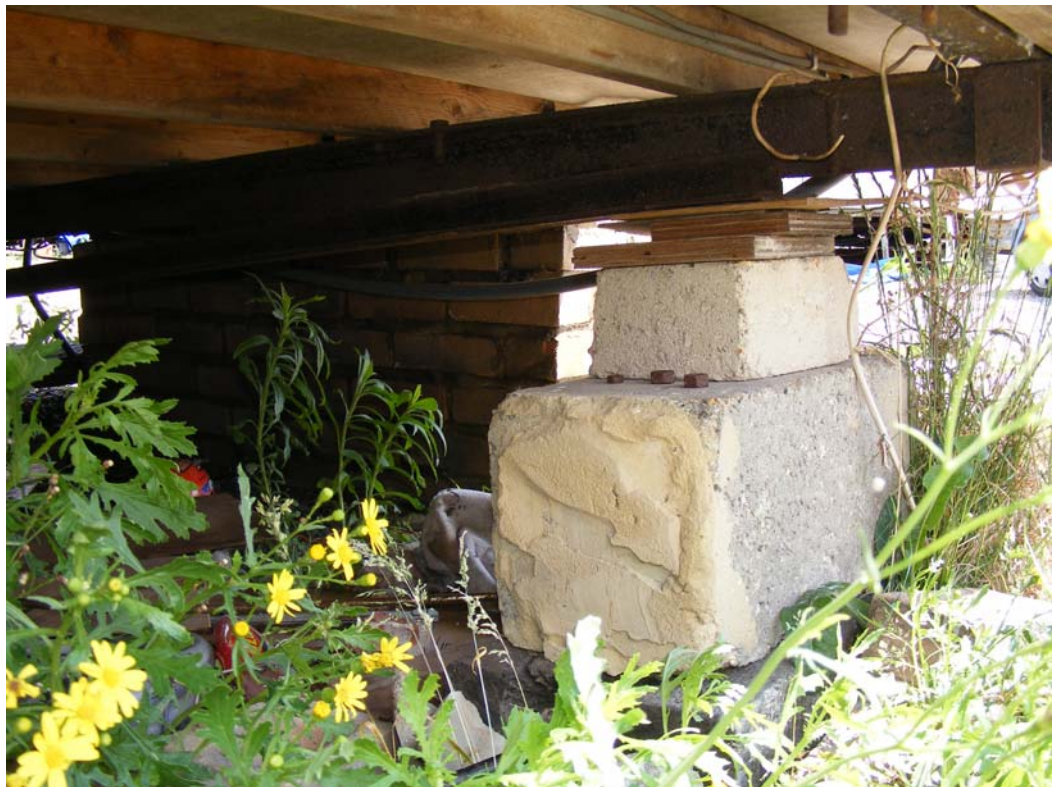
Props can be simple block piers
